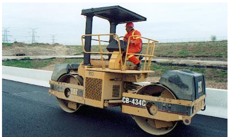
Cat roller on breakdown duty for Gazzola Paving's 407 ETR subcontract.
